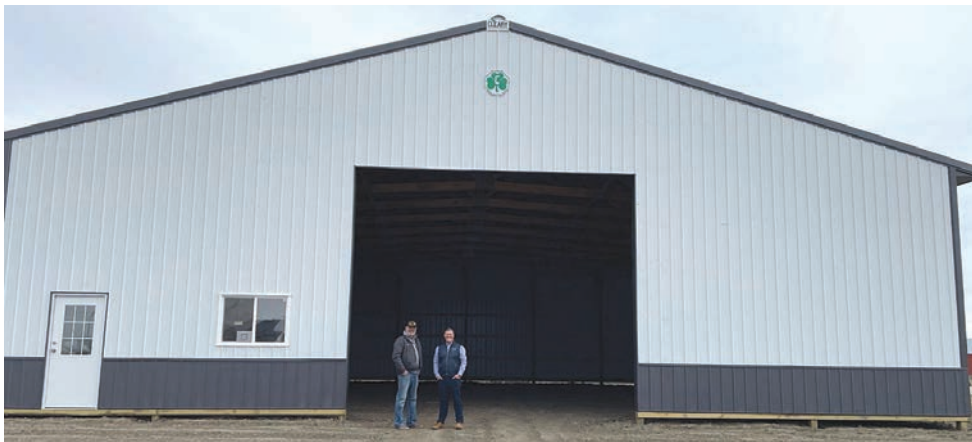
← Shane Davis (operations manager) and Chris Boshart check out the progress on the new seed shed constructed at the Hutchins location.
