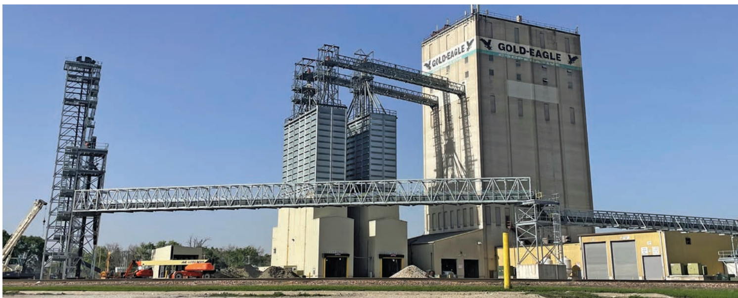
Construction is progressing nicely at the feedmill in Eagle Grove.
